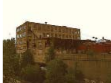
2009 photograph of the Garfield Park site located at N. 31st & Garfield.
